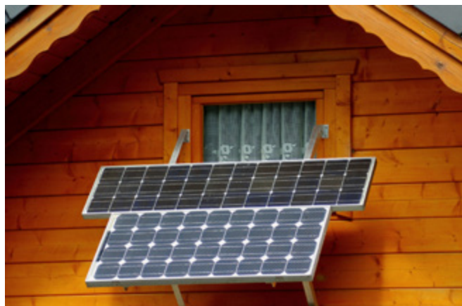
Mini-PV-System – Example
